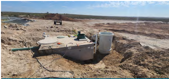
Foreground new 4,000-gal septic tank; background 120 ft by 120 ft evapotranspiration bed, underlain by impermeable liner
