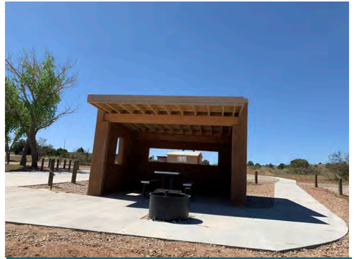
Eastside Campsite Accessibility Upgrade Shelter
