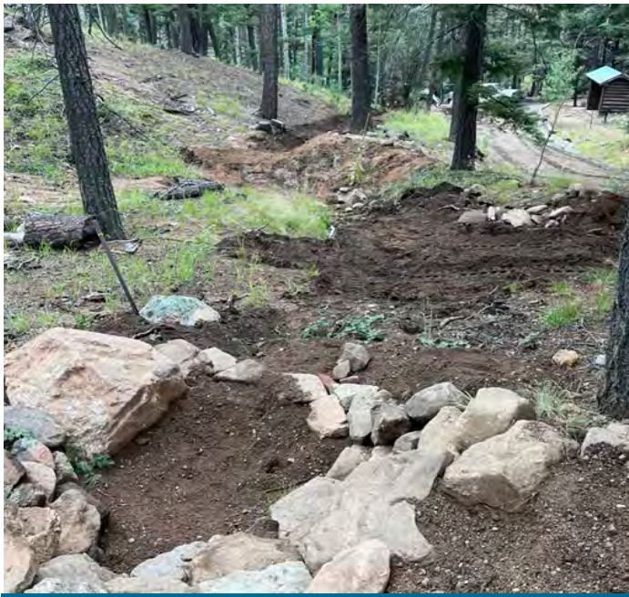
Rock check dams to reduce erosion and increase infiltration of stormwater runoff
