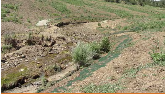
Damage caused by storm in 2013
