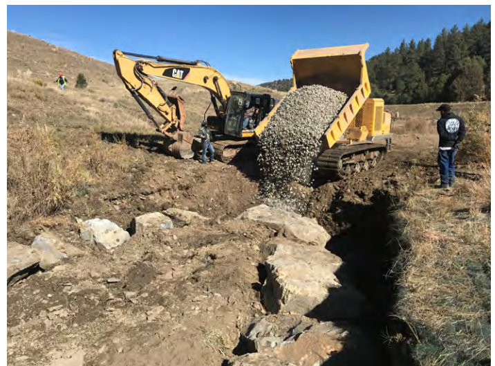
Construction of a cross-vane rock structure at the site, which is an engineered feature designed to create a pool, & slow water flow in the stream channel and prevent erosion.
