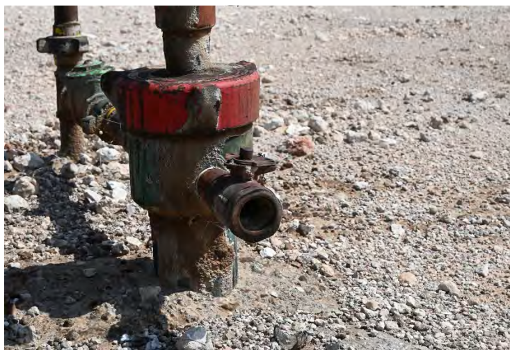
Fig. 4: Photograph of Pumpjack at South Red Lake II Unit #57 (API # 30-015-36116), Charlie Barrett, Aug. 14, 2025.
