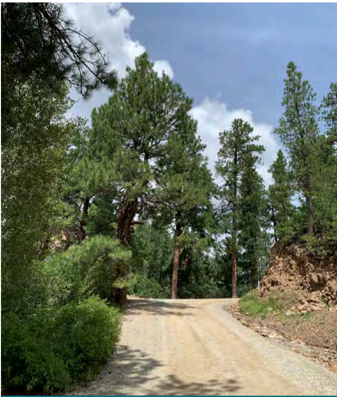
Lake Fork Road Improvements Looking North
