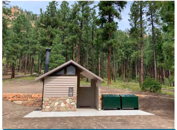
Single vault toilet with sidewalk & trash receptacles
