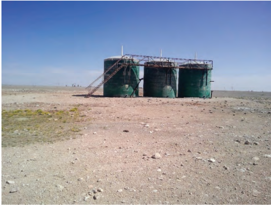
The storage tanks have been removed. Photo depicting condition of the well pad
