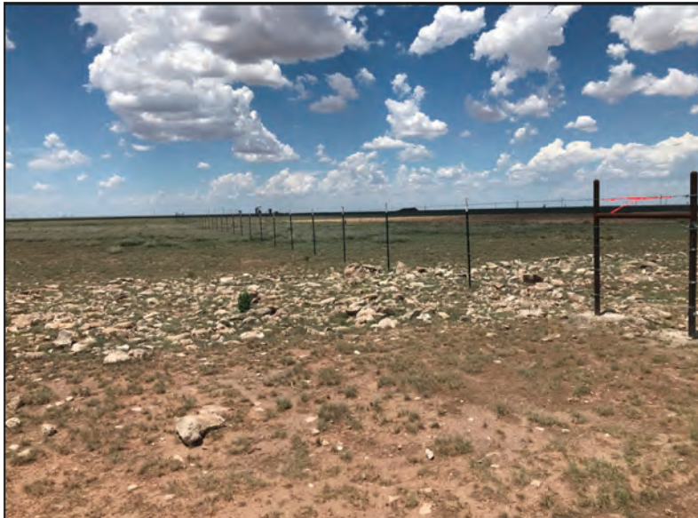
Fencing installed as part of previous project
