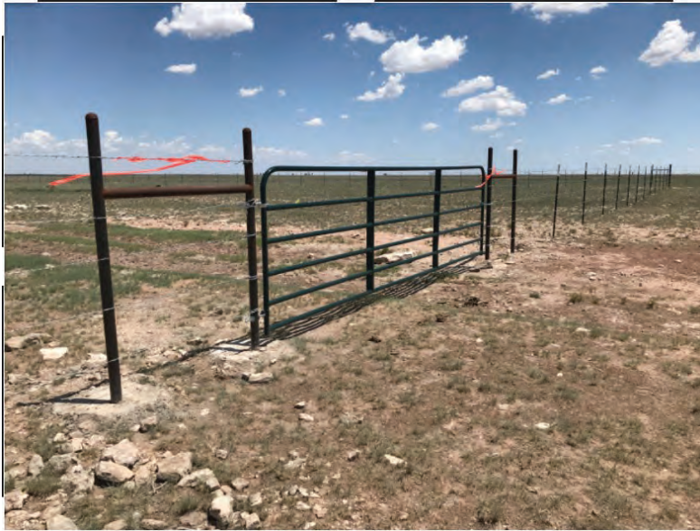
Fencing installed as part of previous project
