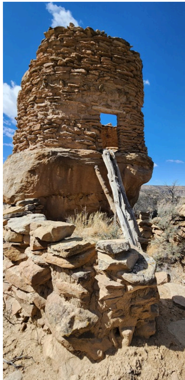
The Cultural Resources Office has partnered with the Navajo Nation to help restore defensive structures like this one.
