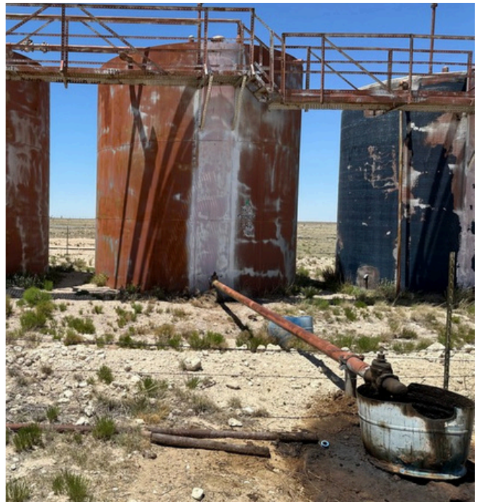
A site on state lands assessed by ECO for cleanup.
