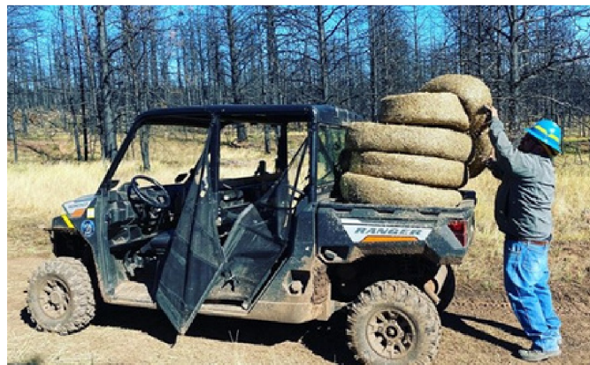
Staff placed straw wattles throughout the Cook's Peak landscape as a post-fire erosion control measure.
