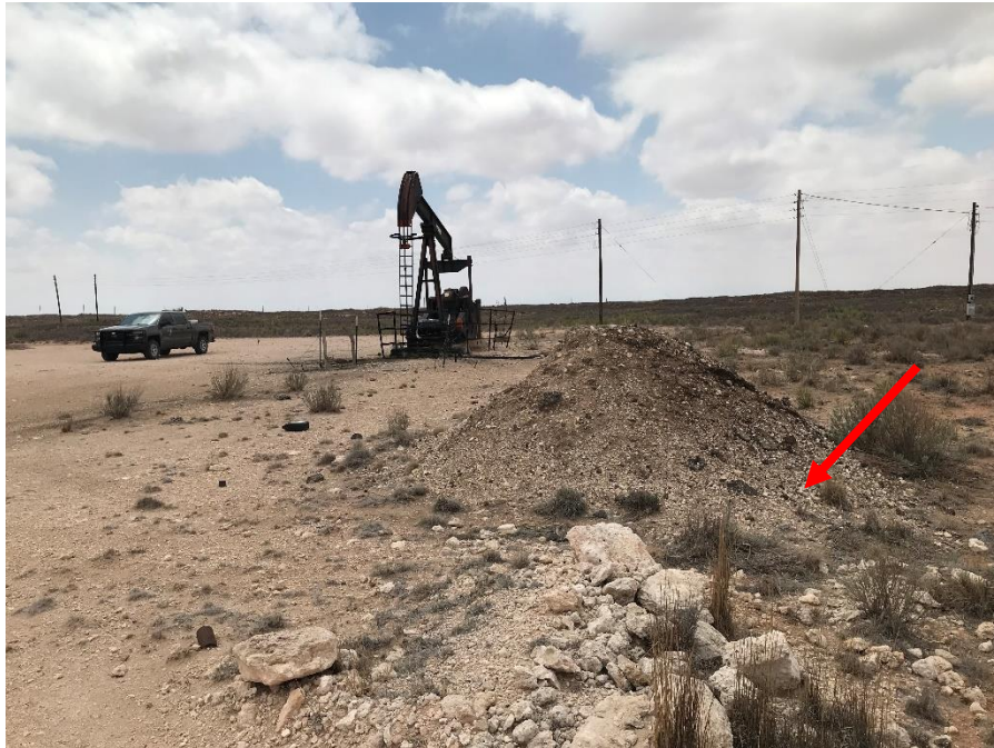
Photo 29: One small stockpile of contaminated soil near the pumpjack (no liner or secondary containment beneath soil).
