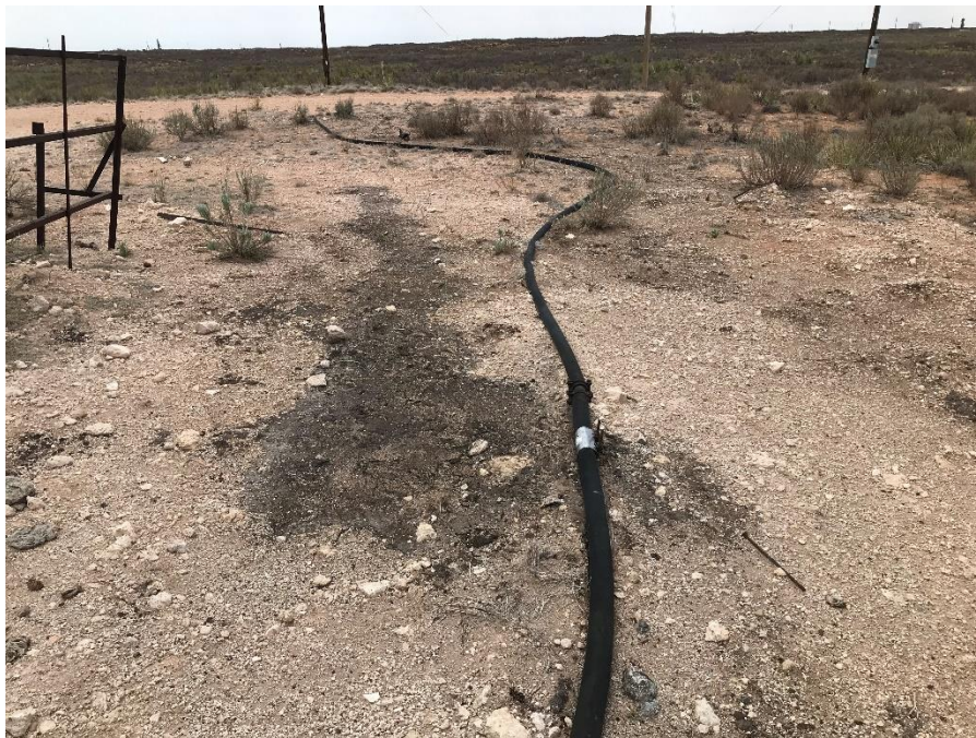
Photo 30: Flowline patch, evidence of prior leak on this pipeline.
