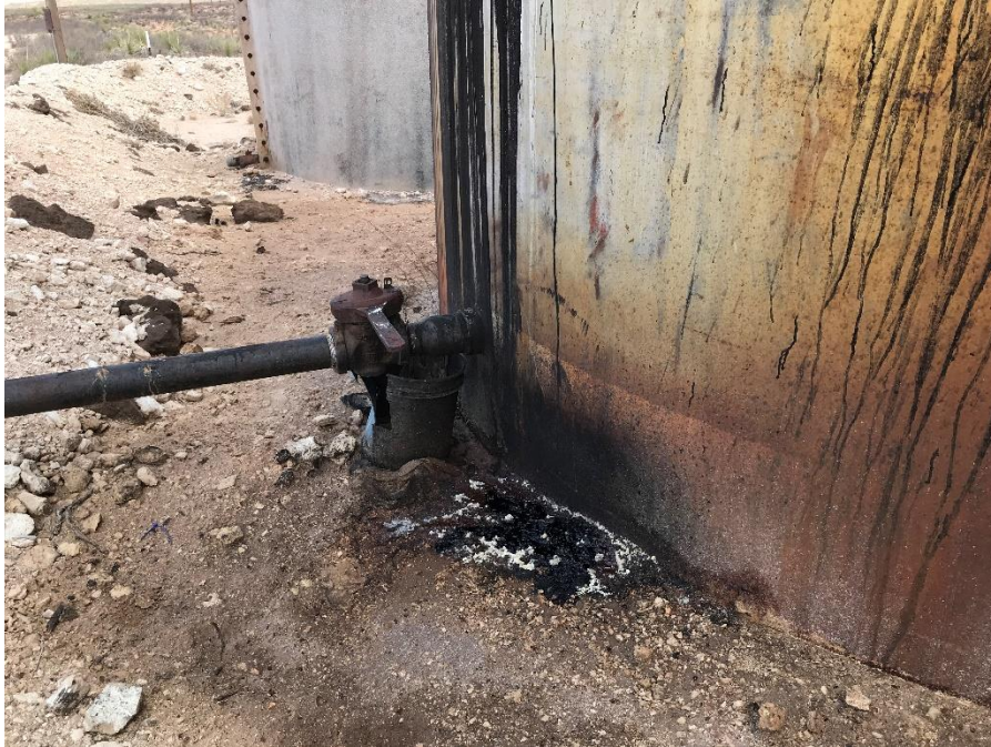
Photo 37: Damaged storage tank and staining at the base.
