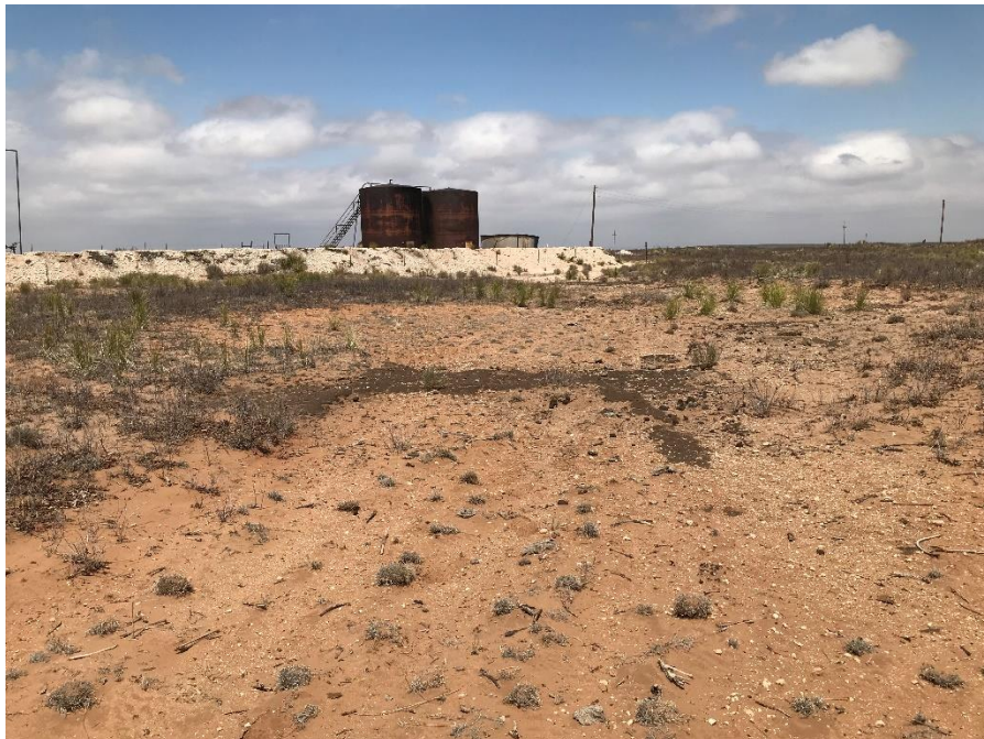
Photo 40: Evidence of previous release (bare soil and asphaltine) observed directly south of the tank battery
