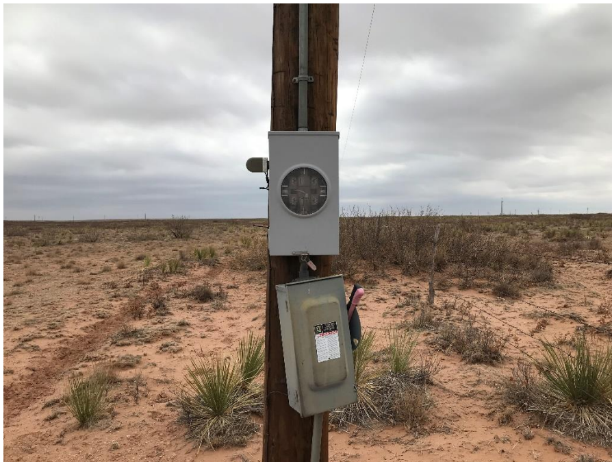
Photo 4: Broken electrical meter observed at the Cato San Andres Unit Well #504.
