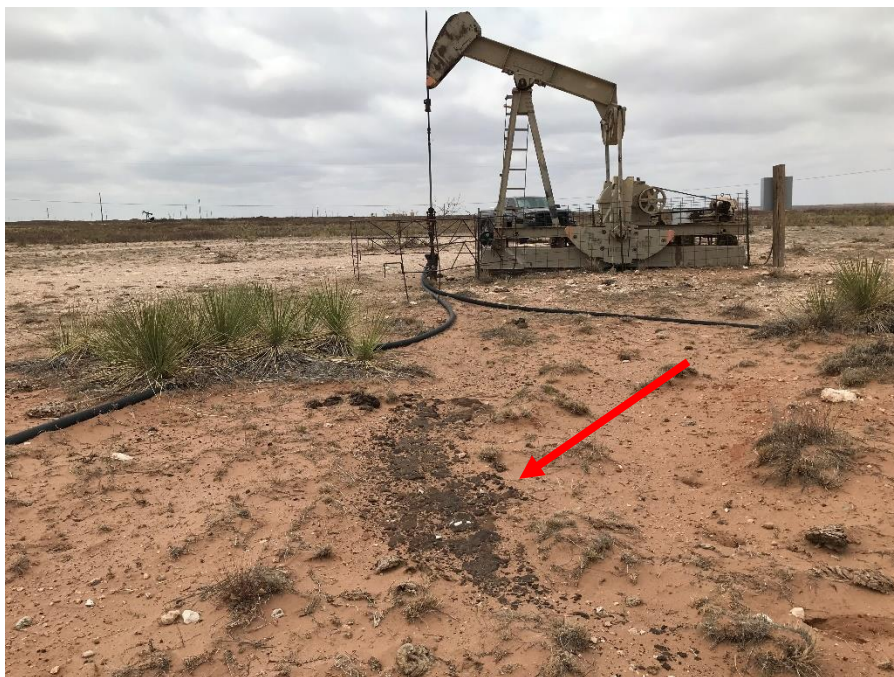
Photo 8: Evidence of a prior release observed near the well's flowlines (NW4/SW4, section 02, T08S, R30E).
