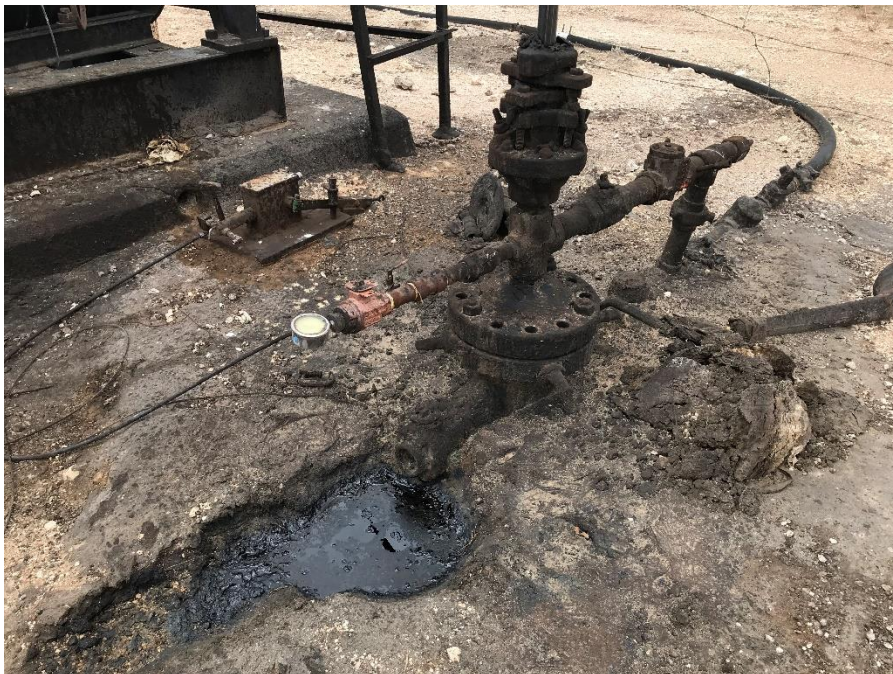
Photo 28: Close up view of the State 32 #003 wellhead, staining present.
