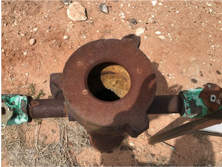
Photo 15: Close up view of unplugged/open wellbore at the Cato San Andres Unit Well #006.
