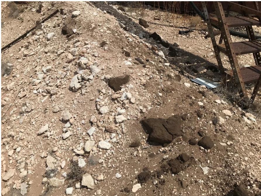
Photo 38: Large clumps of contaminated soil in the containment berm structure.
