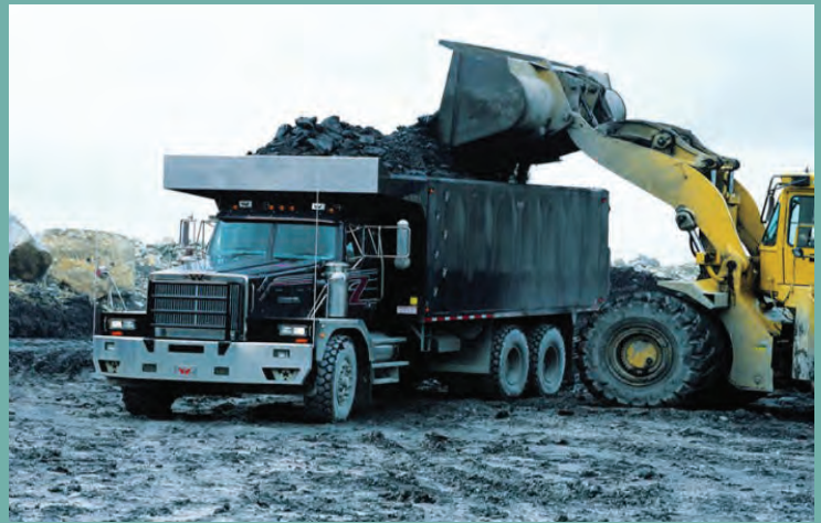
Caliche mining operators load a truck for transport. Caliche is a valuable mineral material used in road base and well pad construction for oil and gas development and leasing activities.
