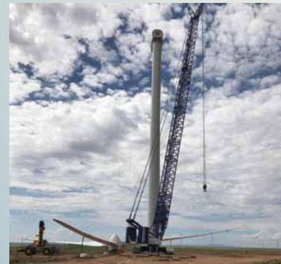
Crews install a wind turbine at El Cabo Wind Project in Torrance County.
