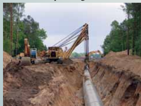
Crews install a 36-inch outside diameter pipeline which bores under an access road in Eddy County.
