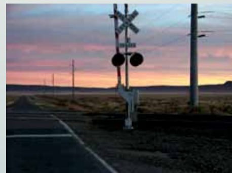
An electric line easement and access road cross State Trust Lands in Torrance County.
