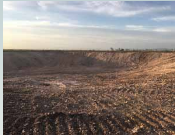
The project site after trash removal includes perimeter fencing provided by project partner Edison Ranch.
