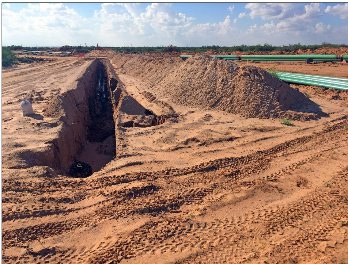
A deep trench was among the surface disturbance at the site in Lea County.
